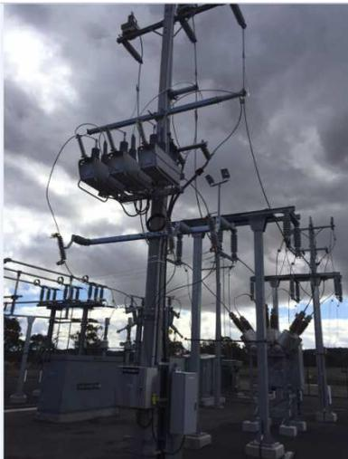
Figure 5 Single Triple Recloser used for faulted phase earthing within a substation in Australia
